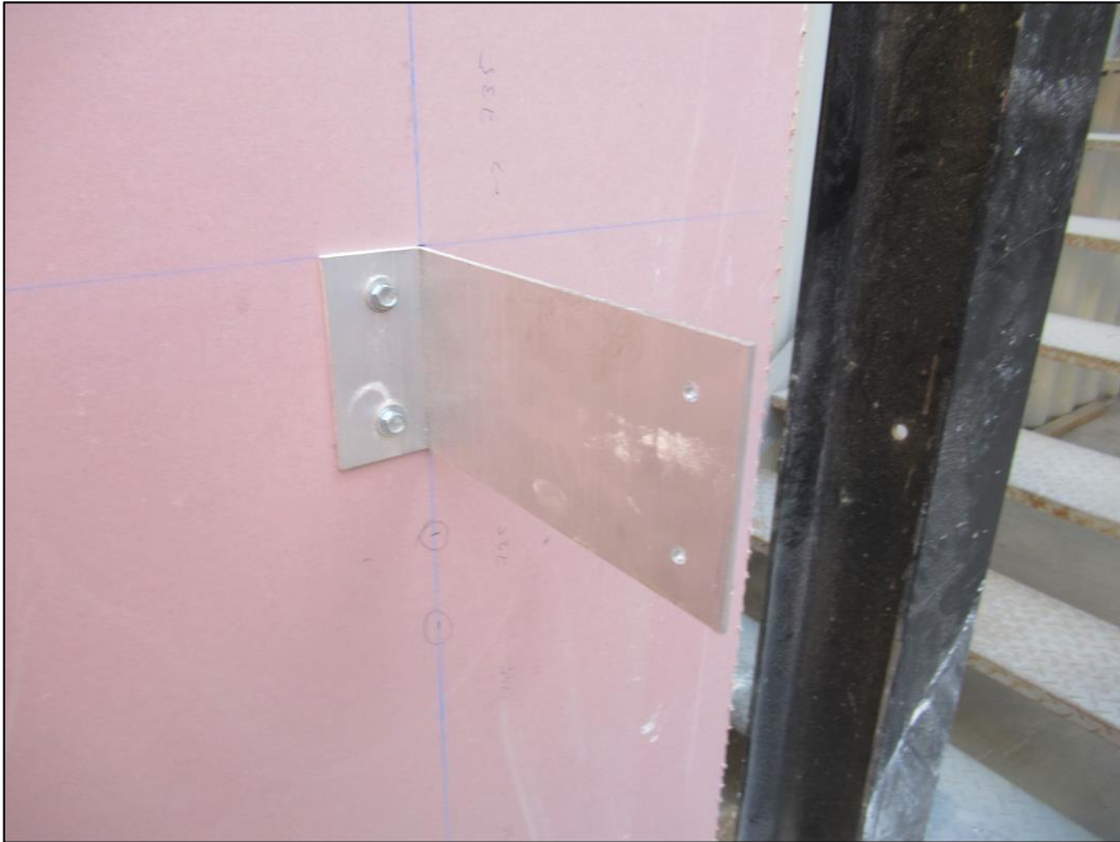
Picture 1: A view of Aluminium Wall bracket fixed to the base wall.
