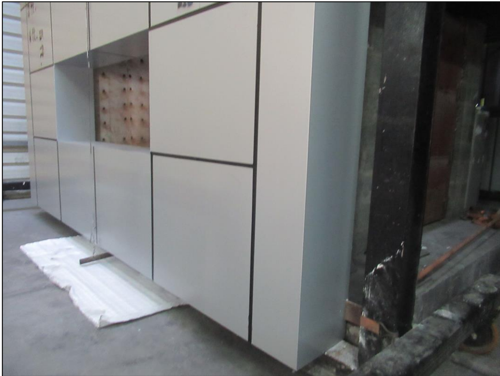
Picture 9: A view of Vertical termination of the system.
