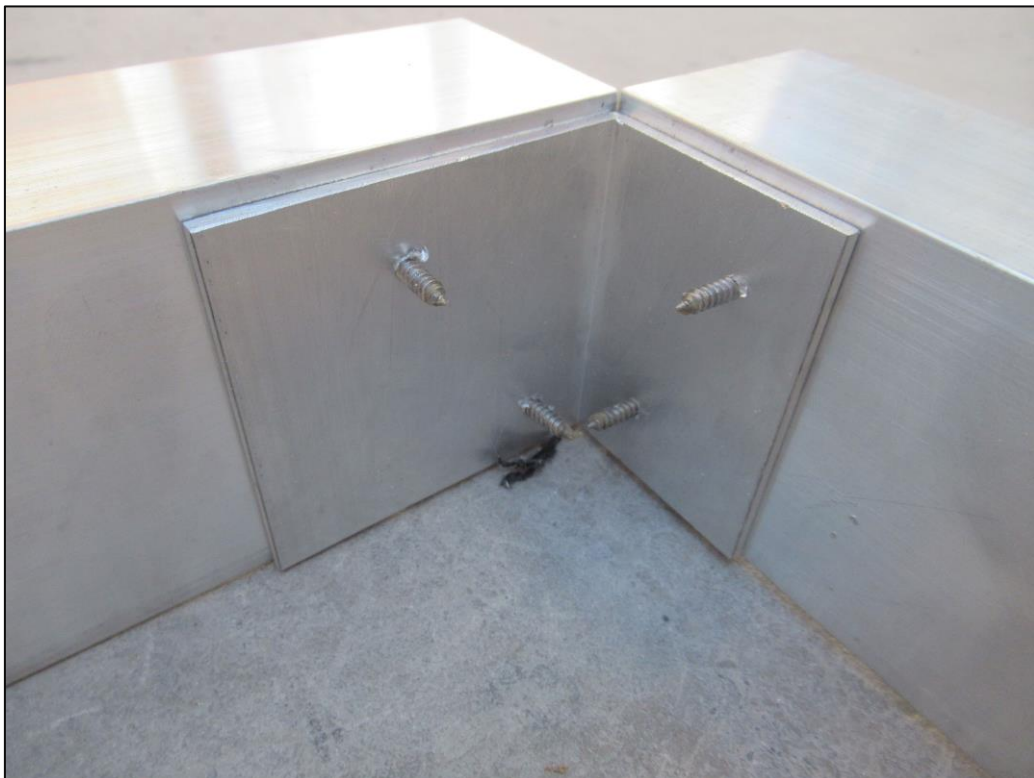
Picture 2: A view of Runner connector used to attach the Vertical Runner to the Horizontal Runner.
