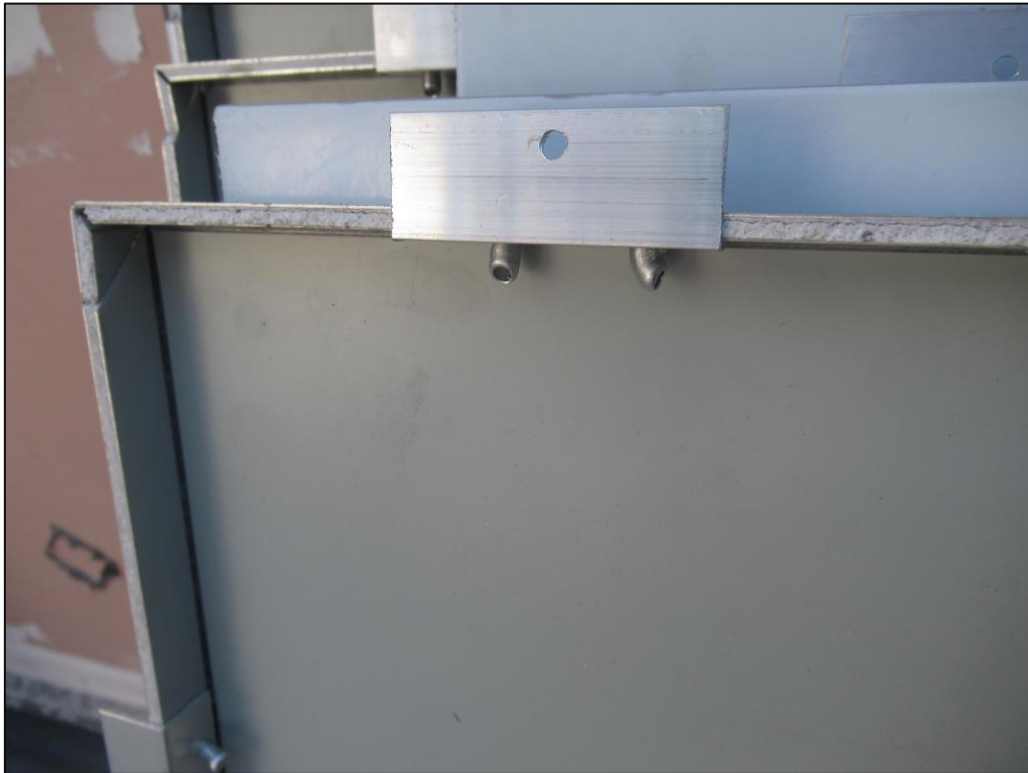
Picture 5: A view of the Prefabricated Aluminium Composite Panel tray profile module.
