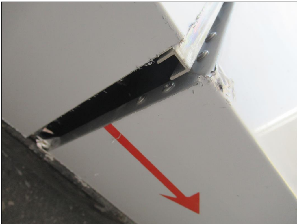
Picture 8: A view of U-Profile fixing in the Panel joint gap.
